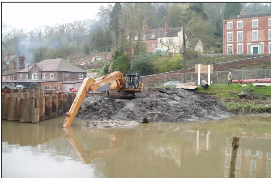
Silt clearance nearing completion
