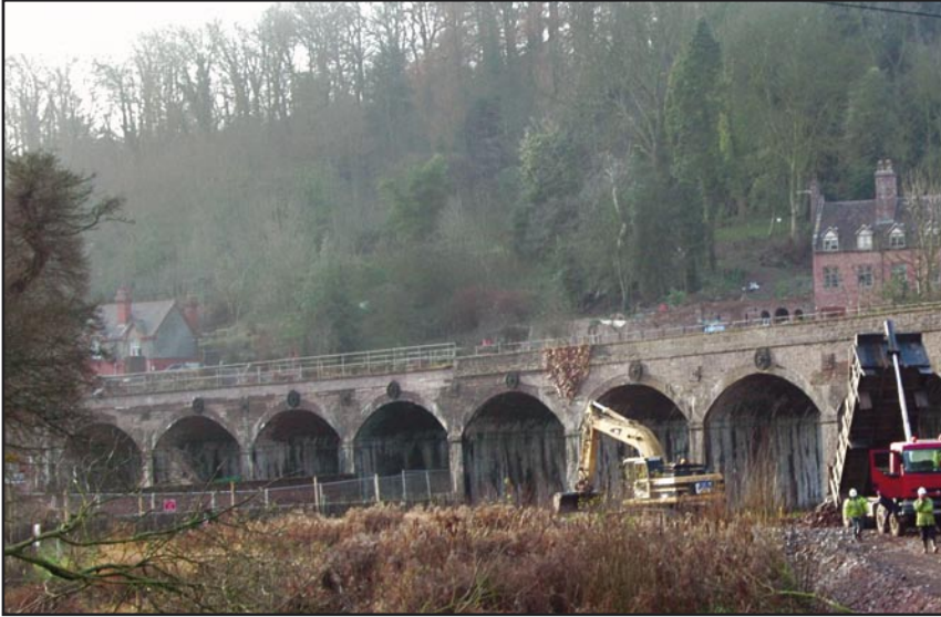
Access road construction underway
