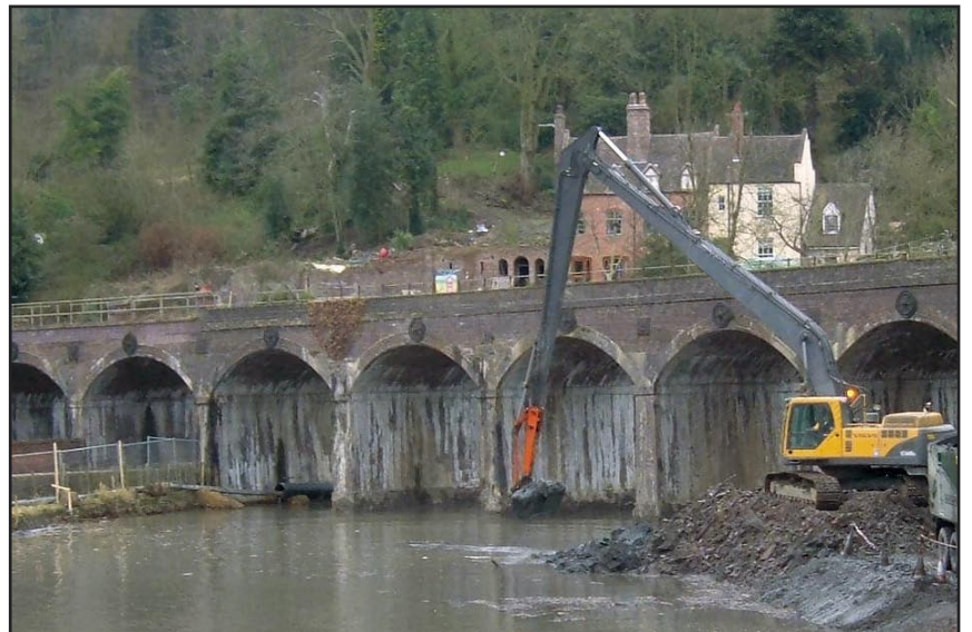
Silt clearance nearing completion
